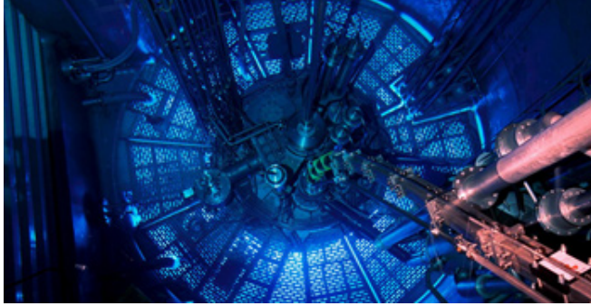
Figure 4.1: Top of the ILL nuclear reactor. The blue light emanating from it is caused by the Cherenkov effect (picture from [61]).
