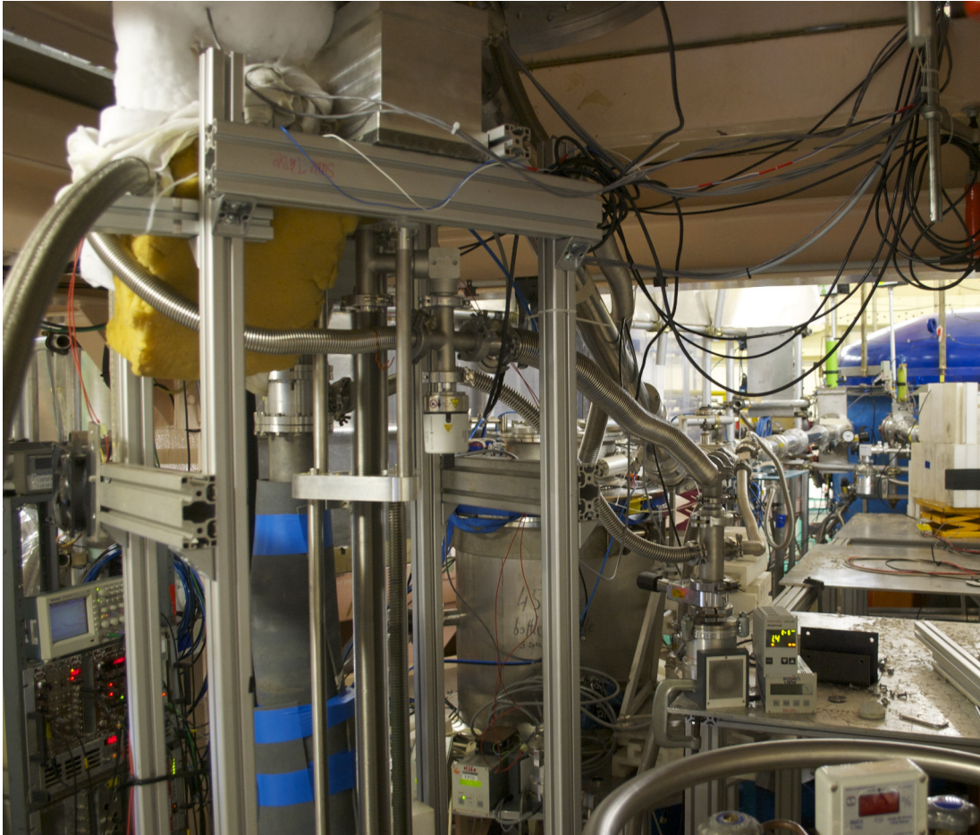
Figure C.2.: Close-up of the mechanics below the cryostat. The big ice block in the upper left corner has formed around the entrance of the LN 2 spirals that are used to cool the permanent magnets. The big aluminum box to its left is the casing of the detector switch and below the switch one can see the mechanics of the Teflon piston. The whole system is connected to a turbo pump sitting on the aluminum table at the lower right corner of the picture and equipped with multiple bypasses in order to avoid dead volumes. In the background we see the blue UCN turbine and the main vacuum shutter of the EDM-beam line. The total guide length from the shutter to the cryostat is about 4 to 5 m.
